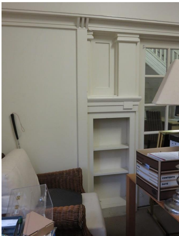
Figure 3.26 The timber joinery adjacent to the door of the office. (Source: GML 2017)
