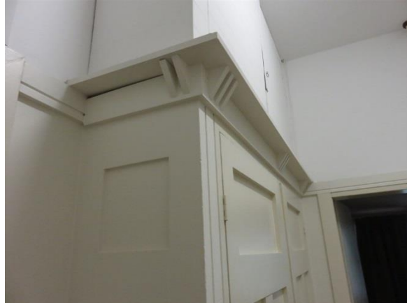
Figure 3.35 The joinery unit in the upper landing, which appears to have been relocated from elsewhere in the building. (Source: GML 2017)
