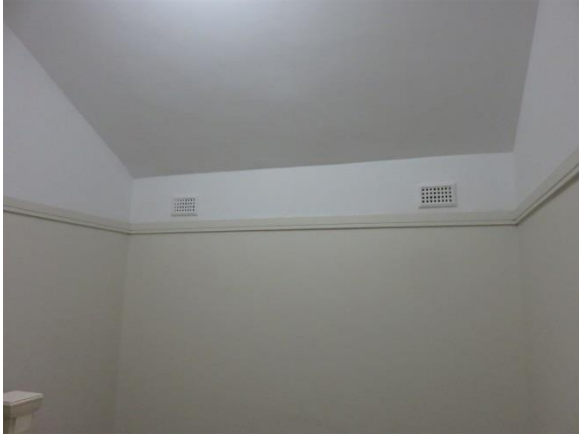
Figure 3.34 The upper part of the eastern wall of the upper landing, above the stair. The air grilles suggest this was originally an external wall. (Source: GML 2017)
