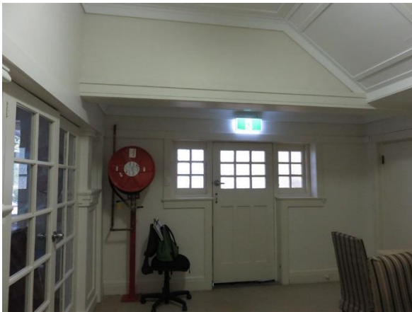
Figure 3.24 The north wall of the entry lobby, with front door and sidelights. (Source: GML 2017)
