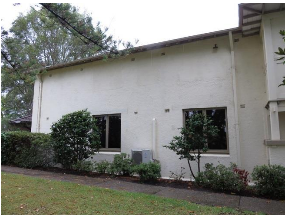
Figure 3.18 The north (front) elevation of the chapel wing. 'Shadows' of former window openings can be seen in the stucco finish. (Source: GML 2017)
