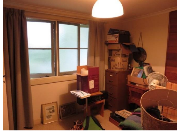
Figure 3.41 The north wall of the storeroom. (Source: GML 2017)
