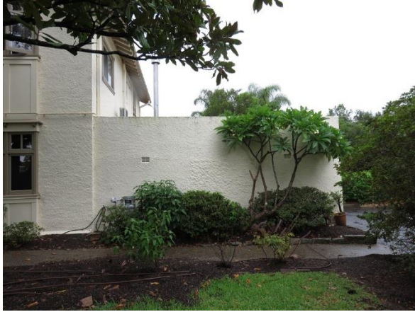
Figure 3.14 The north elevation of the garage. (Source: GML 2017)
