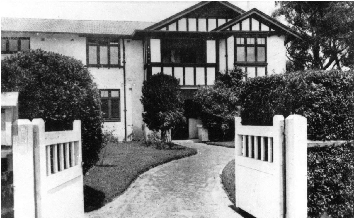
Figure 2.17 c1930 school building and garden path, published Cook, KM 1991, The Railway Came to Ku-ring-gai , Genlin Investments, Pymble. (Source: Ku-ring-gai Historical Society photographic collection)
