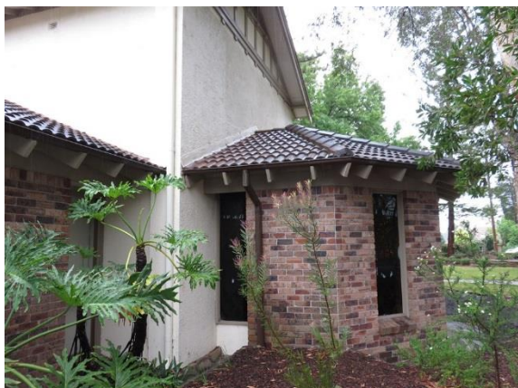
Figure 3.20: The 1980s addition on the eastern side of the chapel wing. (Source: GML 2017)
