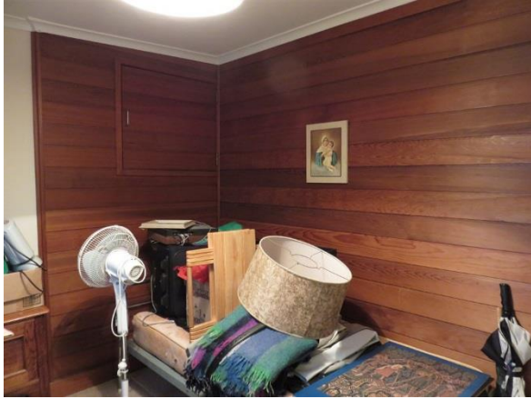
Figure 3.40 The cedar boarding on the south and east walls of the storeroom. The small door in the panelled wall gives access to the chapel's ceiling space. (Source: GML 2017)
