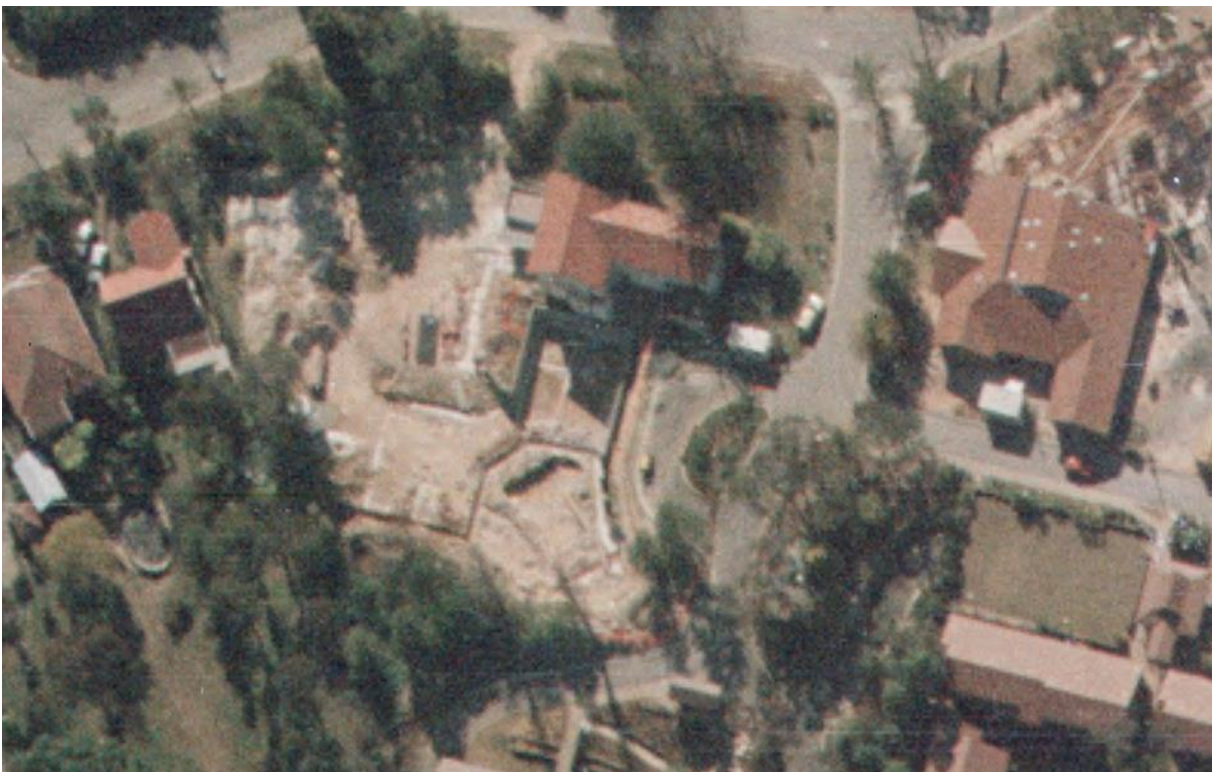
Figure 2.30 Detail of subject site on 1986 aerial showing one of the former school buildings already demolished and the footings of the new administration building. (Source: LPI NSW)
