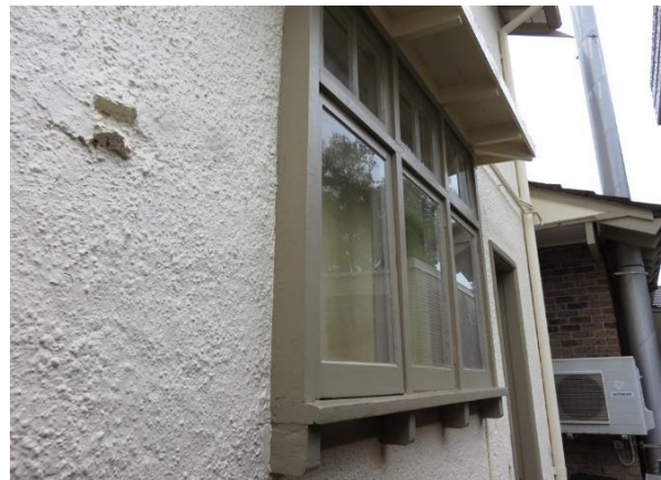
Figure 3.13 Detail of the large timber framed window, west elevation. (Source: GML 2017)
