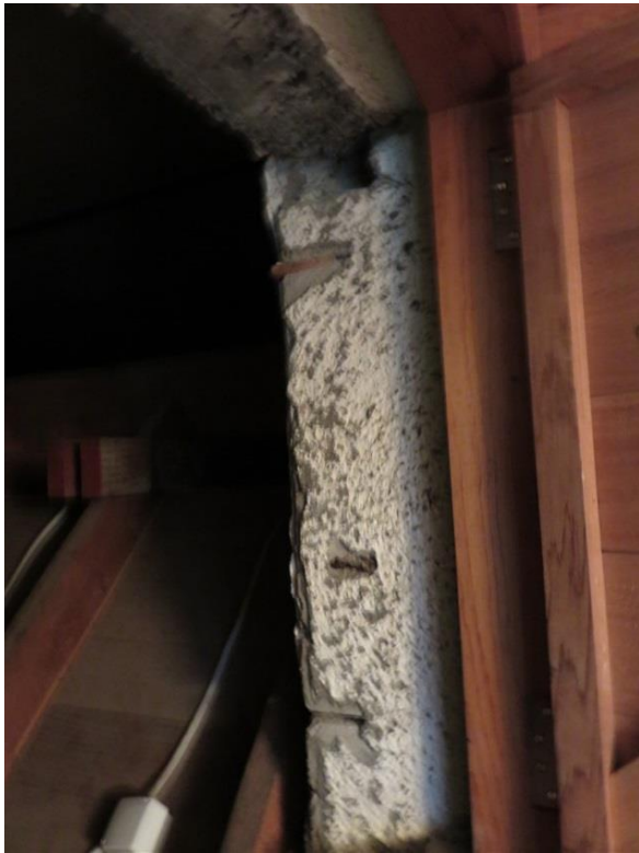
Figure 3.42 When opened the access door allows for views of the building's original external stucco finish and the space above the ceiling of the chapel. (Source: GML 2017)
