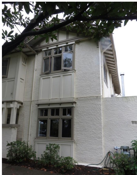
Figure 3.9 The framed wall panels below the windows on the north (front) elevation of Headfort House. (Source: GML 2017)
