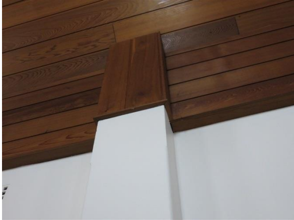
Figure 3.45 A typical wall pier in the chapel. (Source: GML 2017)
