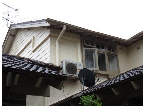
Figure 3.17 The original timber window that exists in the upper part of the east elevation of the main part of the building. The boarded gable of the south elevation can be seen on the left. (Source: GML 2017)
