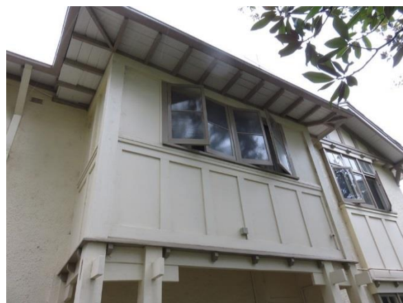
Figure 3.11 The verandah above the entry porch. The windows are a later addition. (Source: GML 2017)
