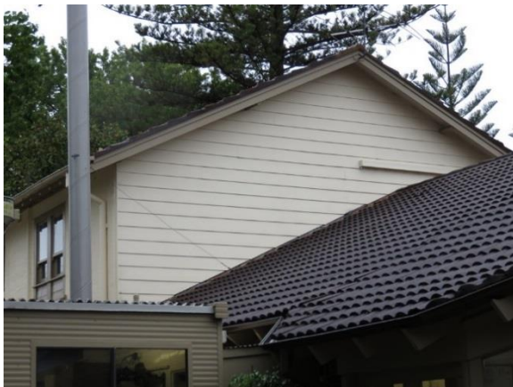
Figure 3.16 The boarded gable is the only part of the south elevation of the main part of the building that is visible. The brown tiled roof in the foreground is part of the 1980s building. (Source: GML 2017)
